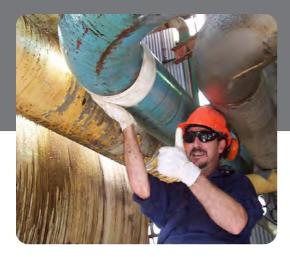
*"Rapp-it is suitable for use on wet or dry pipes. It can even be applied underwater, in fresh or saltwater."*
