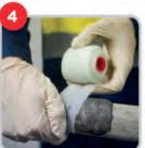
STEP 4: Quickly wrap the bandage around damaged area, extending 50mm (2") either side of the leak. Pull each layer firmly throughout the application. A strong, tight repair is very important.
