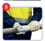
STEP 5: With wet gloves, squeeze the bandage with a rotating motion until resin stops foaming and is set. Allow a minimum of 30 minutes for Rapp-it Bandage to set rock-hard.
