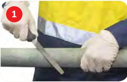
**STEP 1** Shut down pipes or hoses. If pipe cannot be shut down, reduce pressure as low as possible. Apply gloves, then thoroughly clean and roughen the damaged area with a metal file or a wire brush. This helps result in a successful repair.
