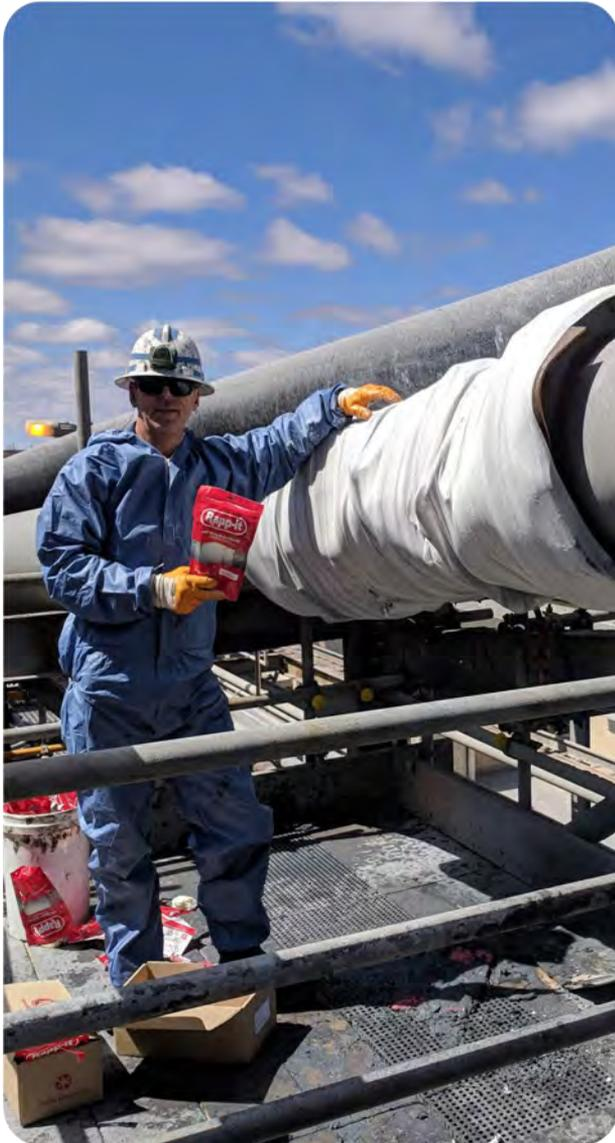
Rapp-it is the Ultimate Pipe Repair System for your temporary emergency pipe repair needs. It is simple to use, with no mixing or measuring required. A successful pipe repair can be achieved in only 30 minutes.
