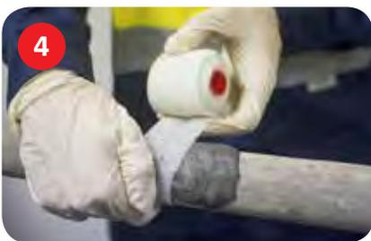
**STEP 4** Quickly wrap the bandage around damaged area, extending 50mm (2") either side of the leak. Pull each layer firmly throughout the application. **A strong, tight repair is very important.**
