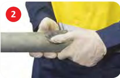
**STEP 2** Tear off adequate amount of Steel Putty. Twist and knead Steel Putty until it is a uniform grey colour and apply firmly into damaged area. Putty will become hot. The putty has a 2-5 minute work life, and the bandage application must begin during this time.
