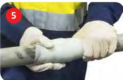
**STEP 5** With wet gloves, squeeze the bandage with a rotating motion until resin stops foaming and is set. Allow a minimum of 30 minutes for Rapp-it Bandage to set rock-hard.
