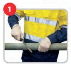
STEP 1: Shut down pipes or hoses. Apply gloves, then thoroughly clean and roughen the damaged area with a metal file or wire brush. This helps result in a successful repair.
