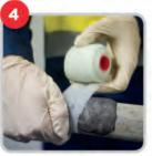
STEP 4: Quickly wrap the bandage around damaged area, extending 50mm (2") either side of the leak. Pull each layer firmly throughout the application. A strong, tight repair is very important.
